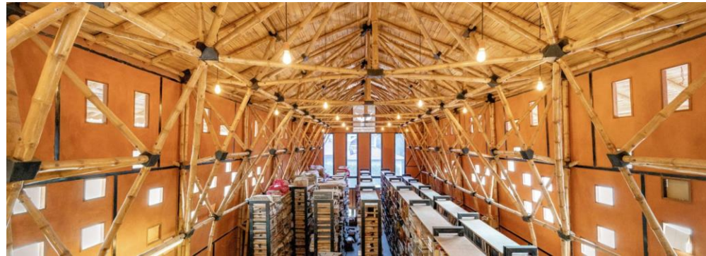
Madan Pustakalaya –(Bamboo Rammed Earth) Abari
