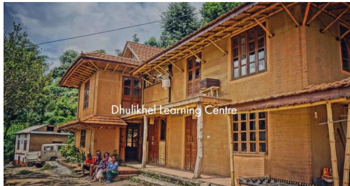
Dhulikhel Learning center –(Bamboo Rammed Earth) Abari
